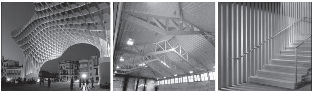
Figure 1. Left: The Construction Metropal Parasol full of LVL ( www.architectureanddesign.com ); middle: long span LVL roof construction ( www.hochstrate.de ); right: LVL as no load bearing material ( www.pinterest.com )
